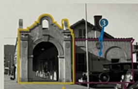
North Facade | Fachada Norte
