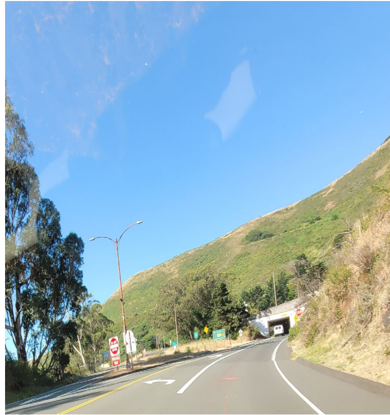
Alexander Ave Looking West at Hwy 101 North On-Ramp and Tunnel to Hwy 101 South
