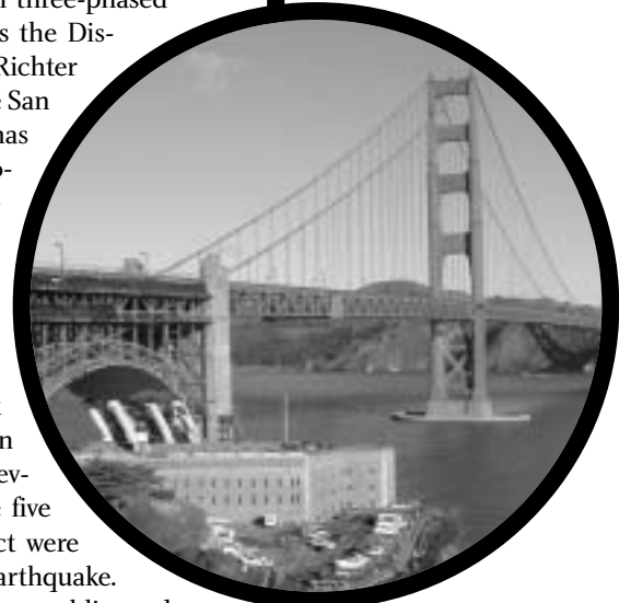
ABOVE: The most complex of the three construction phases is underway and includes the retrofit of the Fort Point arch which is situated directly over Historic Fort Point.
