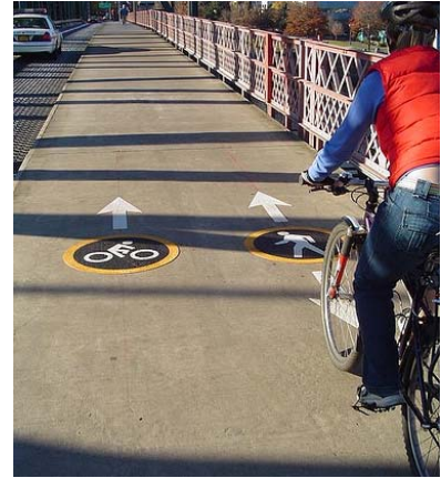
Figure 20 One-way markings on the Hawthorne Bridge, Portland, OR
