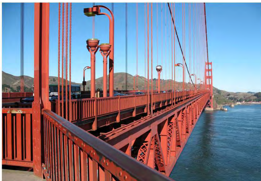
Viewpoint 14 – Bridge Tower
