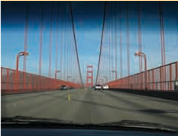
ALTERNATIVE 2A Replace Outside Handrail with Vertical System (see description on page 7)
