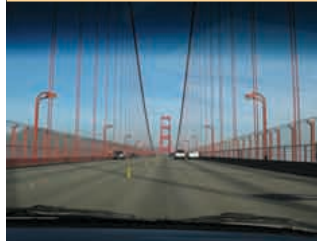
ALTERNATIVE 2B Replace Outside Handrail with Horizontal System (see description on page 7)
