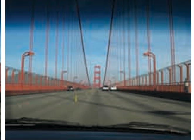
ALTERNATIVE 1B Add Horizontal System to Outside Handrail (see description on page 6)
