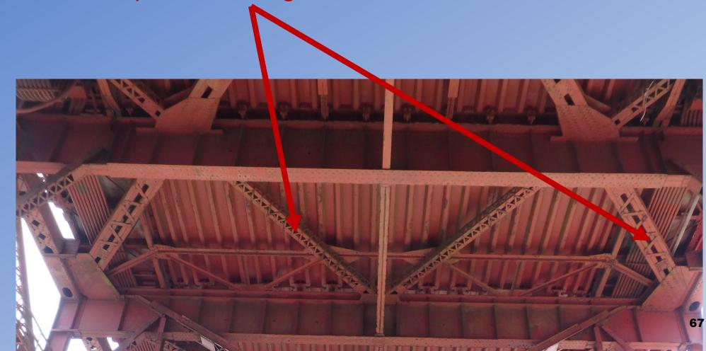
Remove existing center struts between floorbeams at alternate bays
