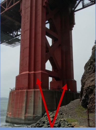
Strengthen existing North and South Tower shafts at base
