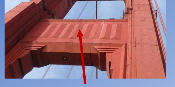
Repair existing North and South Tower transverse cross strut steel façade covers
