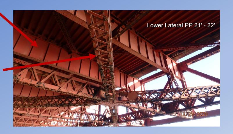
Strengthen existing deck support pedestal connections
